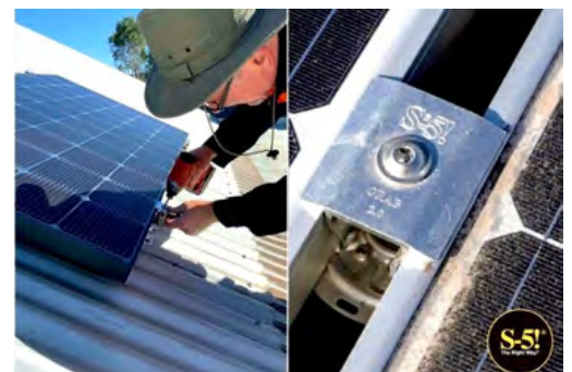
Roof-parallel installation, crosswise to the seam, with the S-5!® PV-Kit 2.0 MidGrab: can be used universally as end and middle clamp.
