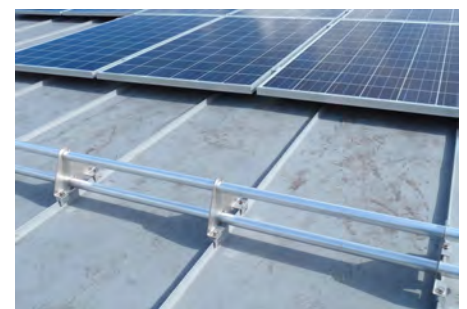
RoofTech Double Tube Holder strong fixed on S-5!® E-Mini clamps
