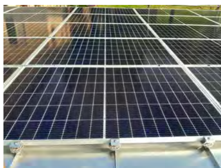
Roof-parallel installation, crosswise to the seam, with the S-5!® PV-Kit 2.0 MidGrab: can be used universally as end and middle clamp.
