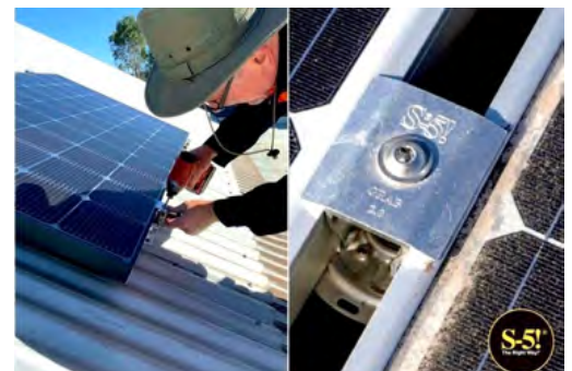
Roof-parallel installation, crosswise to the seam, with the S-5!® PV-Kit 2.0 MidGrab and E-Mini on a double standing seam roof: universally usable as end and middle clamp.
