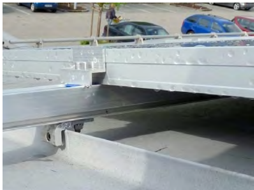
Rail systems fixed with S-5!® E-Mini-FL on a double folded seam roof and with N1.5-Mini on a Nailstrip seam roof.
