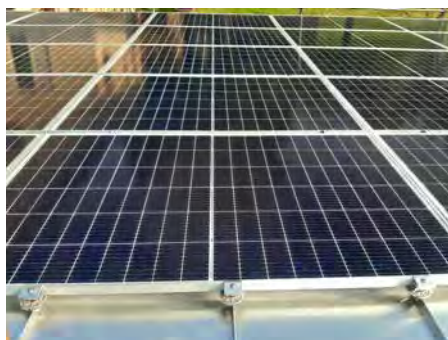
Roof-parallel installation, crosswise to the seam, with the S-5!® PV-Kit 2.0 MidGrab and E-Mini on a double standing seam roof: universally usable as end and middle clamp.
