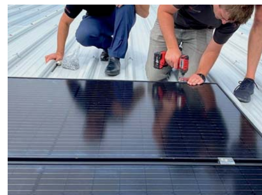
The MidGrab module clamp can be used as Middle- and End-Clamp.
