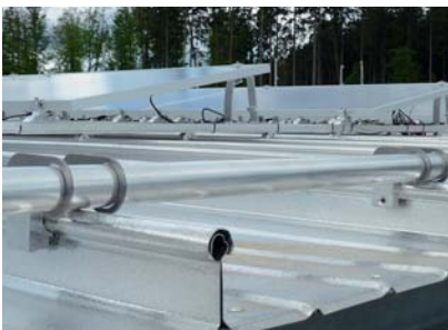
Single-Tube holder on S-5! Z-Mini clamp for round bulb seam
