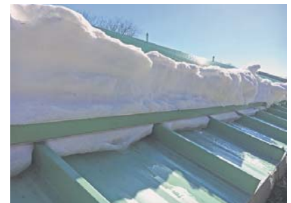
S-5!® ColorGard® mounted on S-5!® clamps with two set screws
