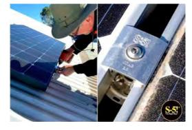
The S-5-PVKIT® 2.0 is mounted on the S-5!®-Mini-Clamp suitable for the seam type or on the trapezoidal holder MTH
