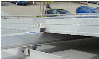
The result of all tests was, with very few exceptions, that the load capacity of each individual S-5!® clamp is stronger than the load capacity of the roof panels or profiled sheets and their attachment to the supporting structure. This applies not only to the Clamps with two setscrews but also to the S-5!® Mini clamps with one setscrew.
