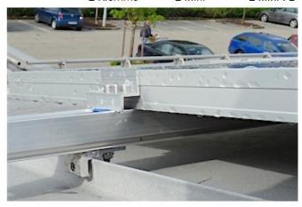
The result of all tests was, with very few exceptions, that the load capacity of each individual S-5!® clamp is stronger than the load capacity of the roof panels or profiled sheets and their attachment to the supporting structure. This applies not only to the Clamps with two setscrews but also to the S-5!® Mini clamps with one setscrew. The loadbearing capacity values from this building approval may be used for static calculations.
