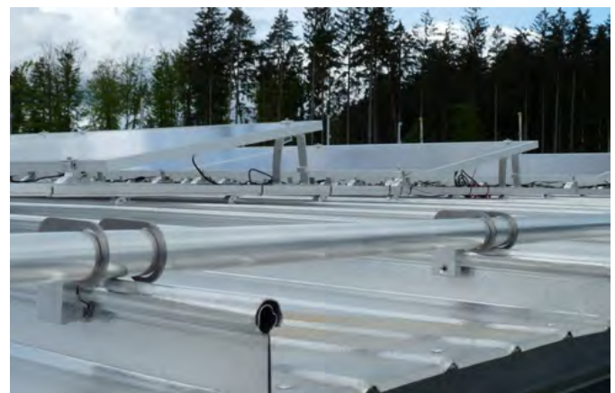
Snow guard on round bulb seam roof with RoofTech Single Tube Holder Type B on S-5!® Z-Mini clamp. Very stable and discreet .
