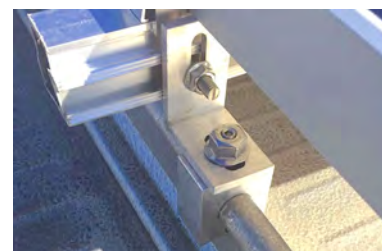
Rail with side screw channel fixed with an angle adapter on S-5!® Z-Mini
