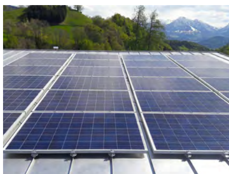
Roof-parallel installation, crosswise to the seam, with the PV-Kit 2.0 MidGrab and E-Mini on a double standing seam roof
