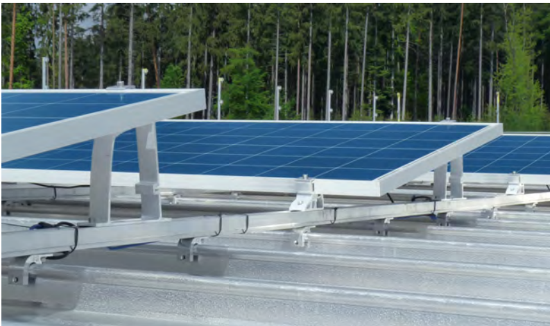
Rail system fixed with S-5! Z-Mini-FL clamps on a round bulb seam roof. Direct Mounting with S-5! PV-Kit 2.0 MidGrab
