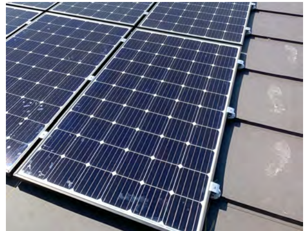
Rail system fixed with S-5! Z-Mini-FL clamps on a round bulb seam roof. Direct Mounting with S-5! PV-Kit 2.0 MidGrab
