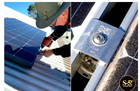
S-5!® PV-Kit 2.0 MidGrab can be universally mounted as middle and end clamp.
