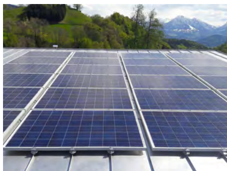
Roof-parallel installation, crosswise to the seam, with the PV-Kit 2.0 MidGrab and E-Mini on a double standing seam roof
