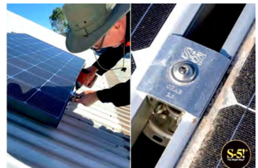
Roof-parallel installation, crosswise to the seam, with the S-5!® PV-Kit 2.0 MidGrab and E-Mini on a double standing seam roof: universally usable as or and middle clamp.
