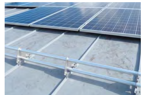
Double Tube holder strong fixed on S-5!® E-Mini clamps
