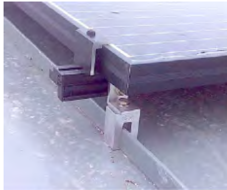
Rail systems fixed with S-5!® E-Mini-FL on a double folded seam roof and with N1.5-Mini on a Nailstrip seam roof.
