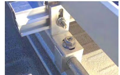
Rail with side screw channel fixed with an angle adapter on S-5!® Z-Mini
