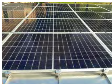
Roof-parallel installation, crosswise to the seam, with the S-5!® PV-Kit 2.0 MidGrab and E-Mini on a double standing seam roof: universally usable as or and middle clamp.
