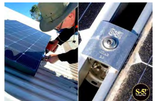
Installation as end and middle clamp
